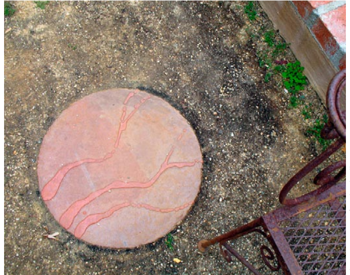
Martin Webb stained over troweled integrally colored skims (overlays) on these mixed-media horizontal and vertical artistic architectural elements.
