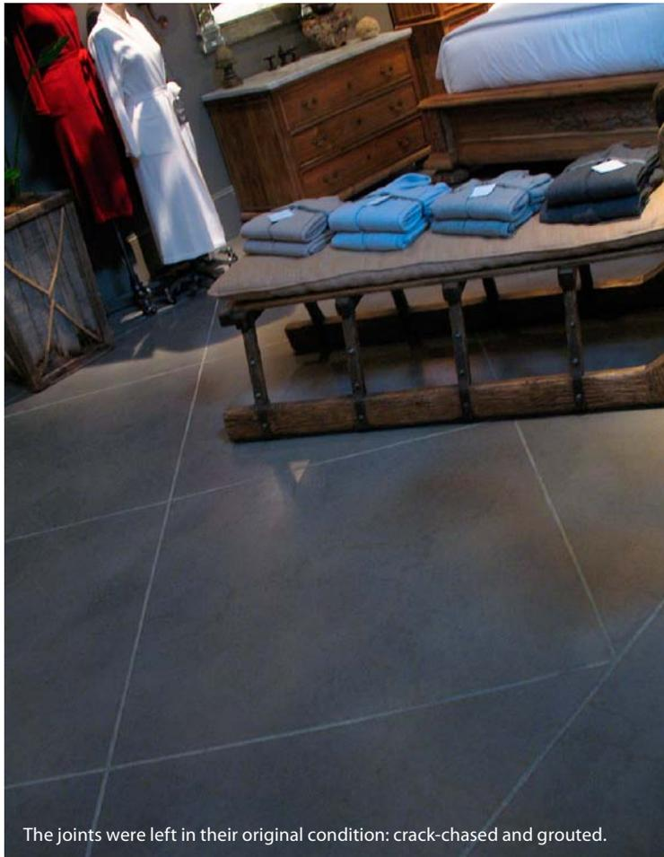
The joints were left in their original condition: crack-chased and grouted.
